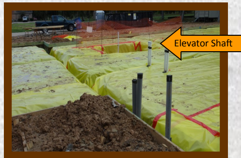
Building Elevator Shaft
