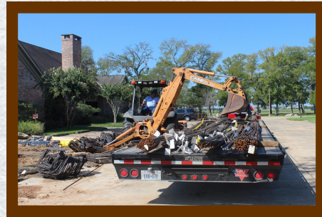
Delivery of Reinforcing Steel for the Slab
